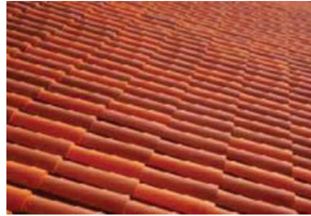
Clay Tile Roof
