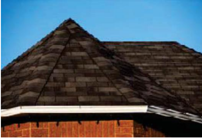
Asphalt Shingle Roof
