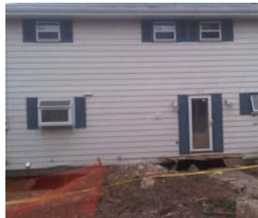
Foundation failure, West Pittston, PA (from FEMA Region III)
