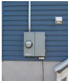
Elevated utilities in Yardley Borough, Bucks County, PA (from FEMA)
