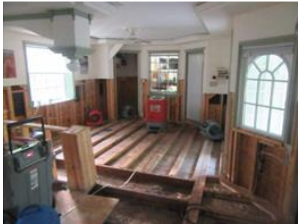
Figure 31. Sleeper System Installed Over a Concrete
